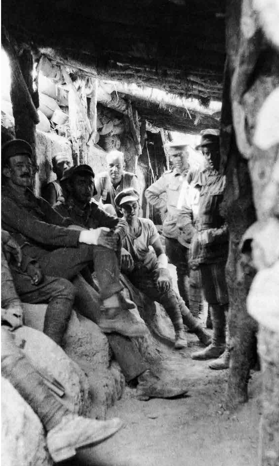
Australian troops rest inside a captured Turkish trench at Lone Pine, 12 August 1915. The overhead covering of heavy pine logs, which made the trenches so difficult to over-run, show evidence of Australian shelling from the attack three days earlier. (AWM G01126)
